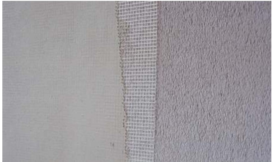
Fig. 17: Fiberglass mesh installation.
