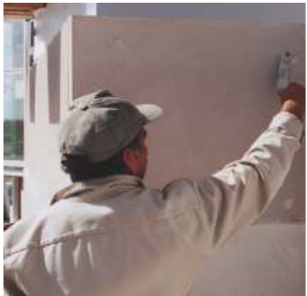
Fig. 10: Patch chips, screws heads and any other imperfections.
