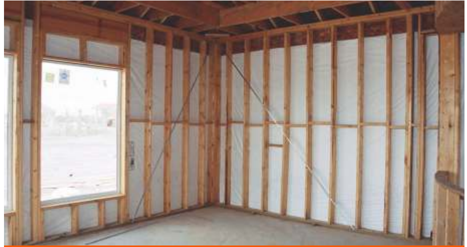
Fig. 5: Interior side of the water-resistant barrier.
