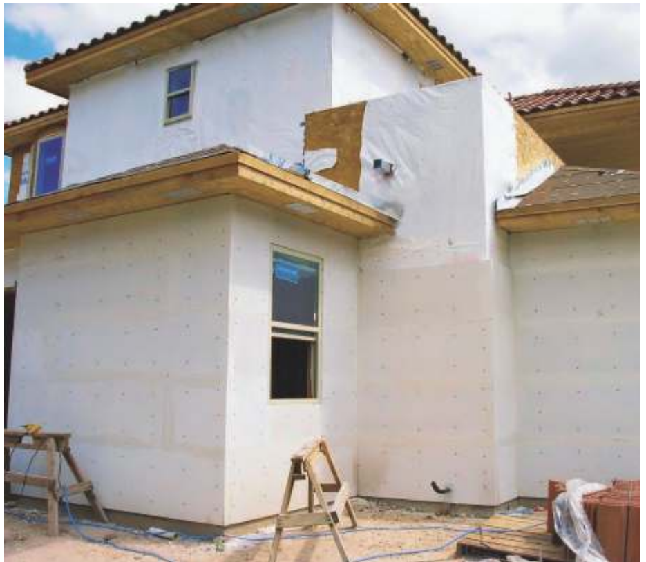
Fig. 15: Hebel® Power Panel on exterior walls.
