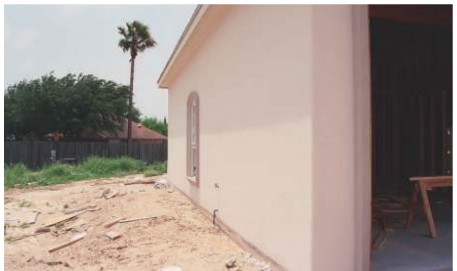
Fig. 18: Finished wall (base-coat and texture).
