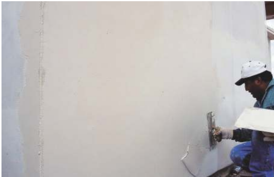
Fig. 16: Base-coat application.
