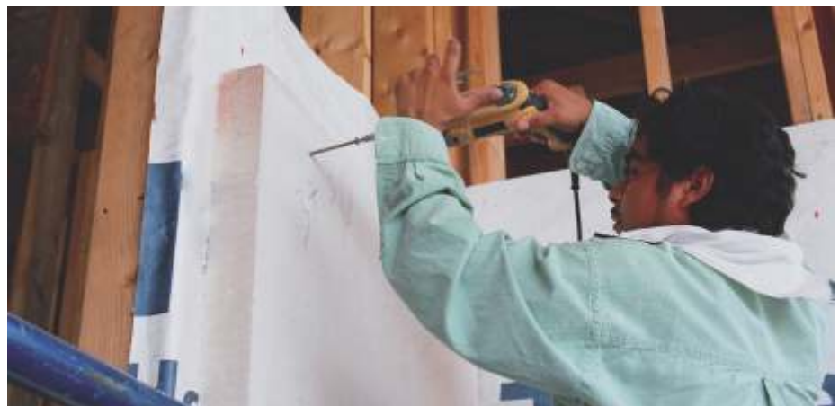
Fig. 7: Use minimum 3 fasteners per stud / board.
