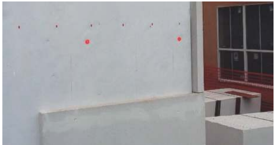
Fig. 6: Overlap Hebel® Power Panel at corners.
