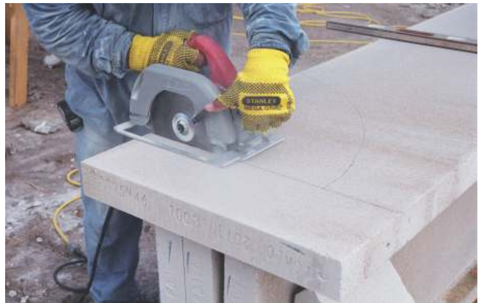
Fig. 5A: Cutting Hebel® Power Floor™ using a circular saw.
