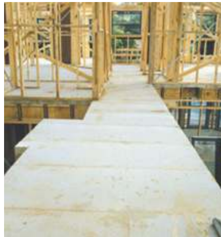
Fig. 7: Fitted Flooring with Internal Loadbearing Wall.
