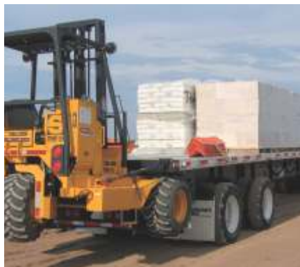
Fig. 5: Forklift and flatbed trailer.
