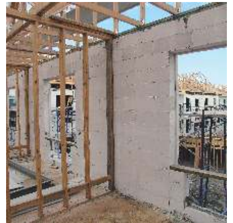
Fig. 21: Construction interior view.
