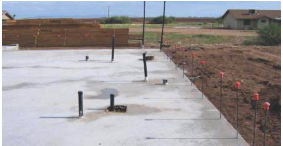
Fig. 6: Check foundation (pipes, drains, reinforcement, etc).
