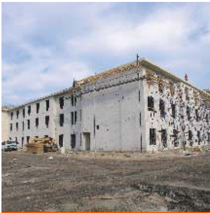
Fig. 22: Three-story hotel construction.
