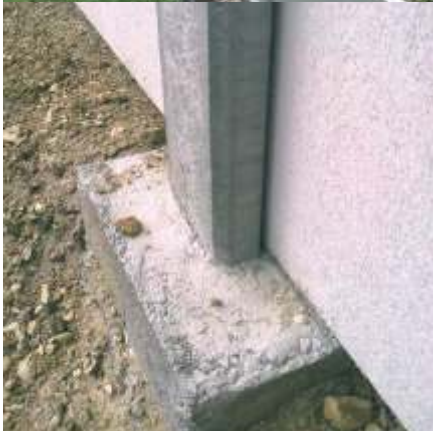
Fig. 6 First Course of Fence Panels.
