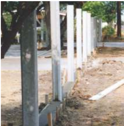
Cast in Place Base
