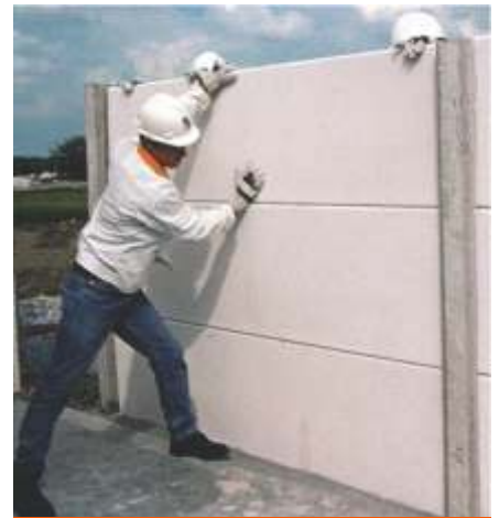
Fig. 7 Hebel® Fence Panel Installation.
